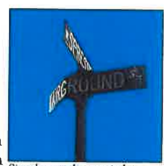
Sign damage due to wind or tearing can mean costly replacements.
