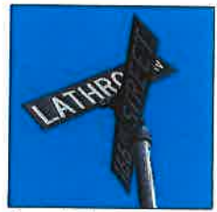
Damaged or leaning signposts are an eyesore in a city's subdivisions.
